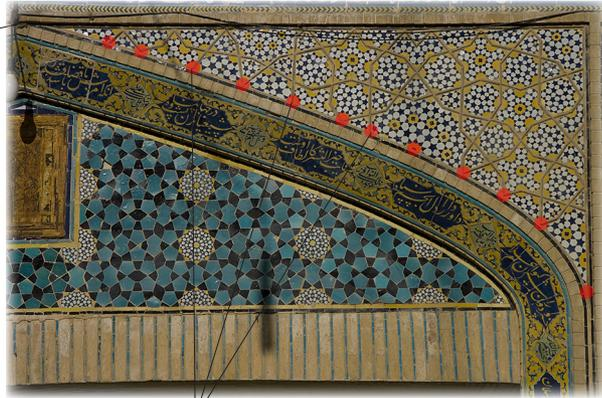
Nodal 'Bézier control points' linking the tiling pattern to the arch geometry
