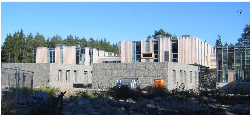
As much as 60% of the external wall is double glazed to maximise the amount of natural light. Half of these are insulated with a semitransparent polycarbonate material called Isoflex, between the layers of glazing. Skylights also contribute to the light airy feel of the building. Parametric modelling was used to find the best ratio between clear glass
