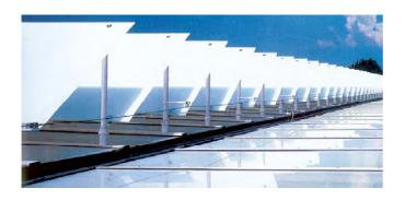
Angled, white enameled glass panels are the uppermost, external shading feature.
