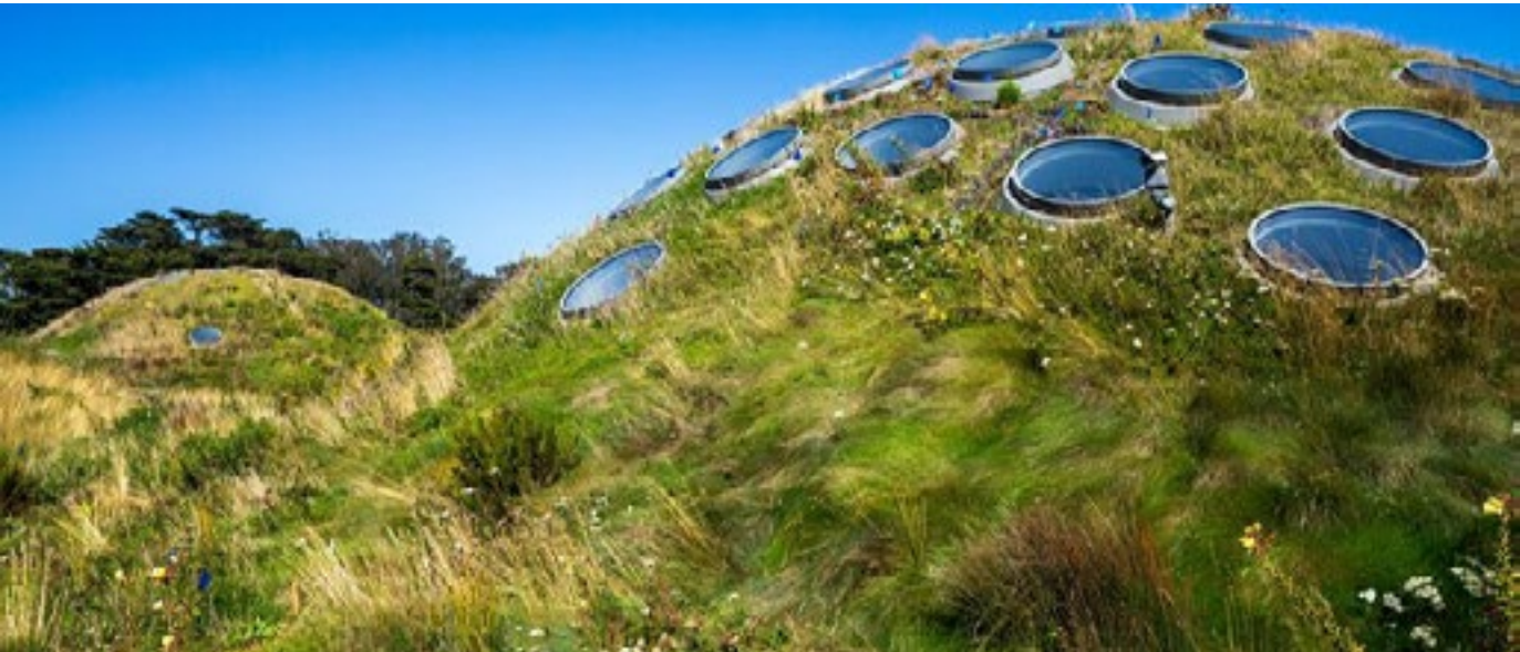
The California Academy of Sciences showcases the potential of living roofs in urban design. With over 1.7 million native plants, the roof provides habitat for local wildlife, improves stormwater management, and reduces energy use, setting a benchmark for sustainable architecture.
