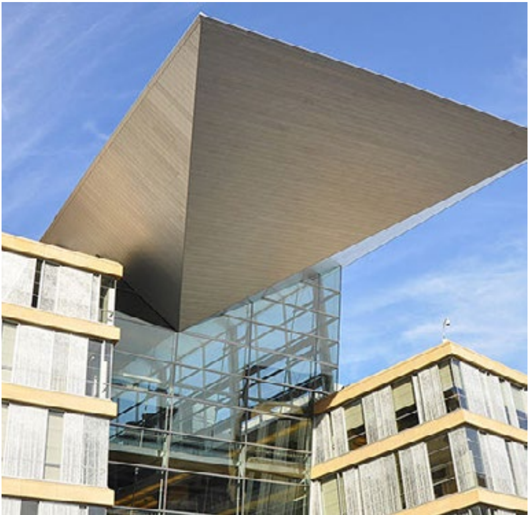
The Minnesota Central Library’s atrium features angled glass, a dramatic architectural feature that reduces reflections of habitat and sky from most angles. The likelihood of fatal collisions at this angle is lessened.
