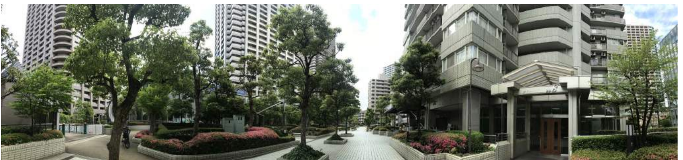
Figure 124: Less than half of the site area has been built up for residential apartments, the majority of the land area has been dedicated to open space or planting, civic and public amenity. This podium level is one storey higher than the main street level.
