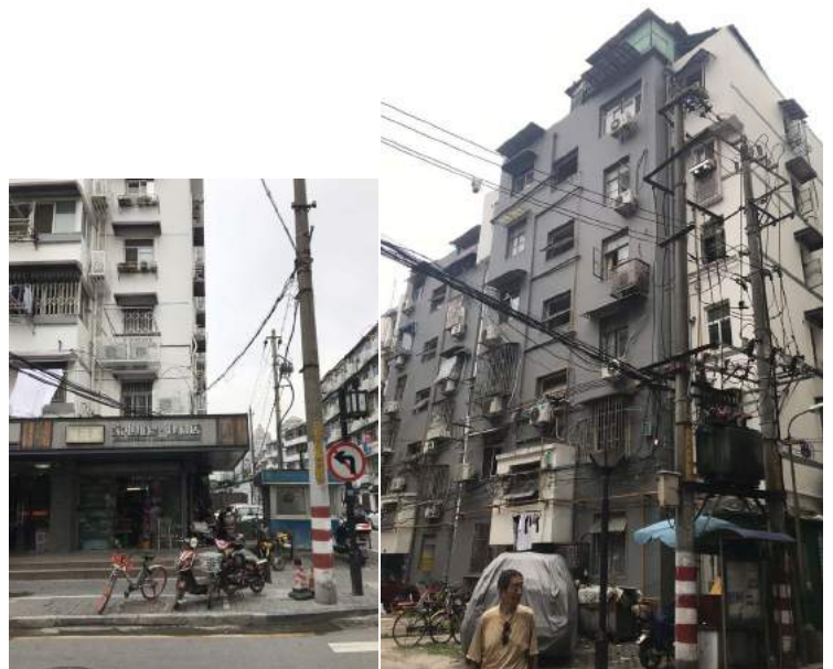
Figure 37: Streetscape along Dasifu Alley, apartment buildings are situated above or behind the shopfronts. These shopfronts become thresholds and interfaces for interaction between the public and private realm.
