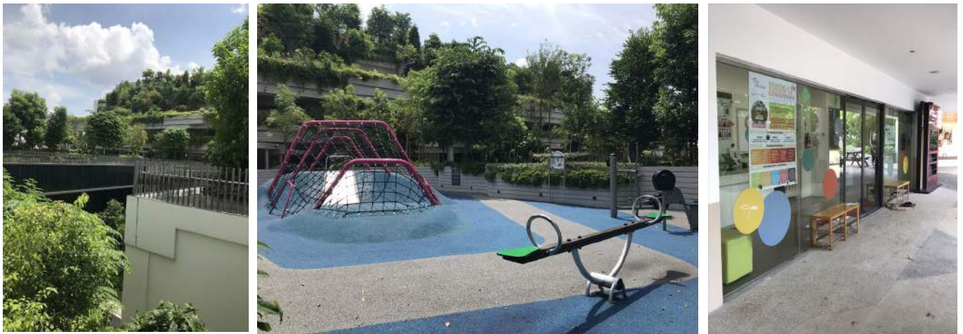
Figure 62: Fourth storey (L5), across the void looking down into the medical centre garden is (middle) the playground between the apartment units and the child care centre (right).
