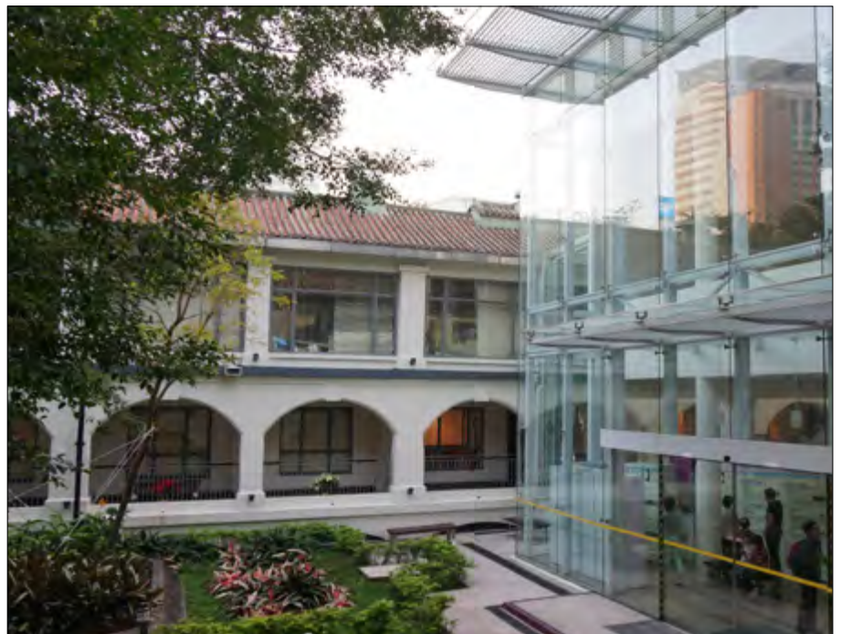
Above Left to Right 03.09 // Steel and glass skylight junction connecting between old and new fabric.
