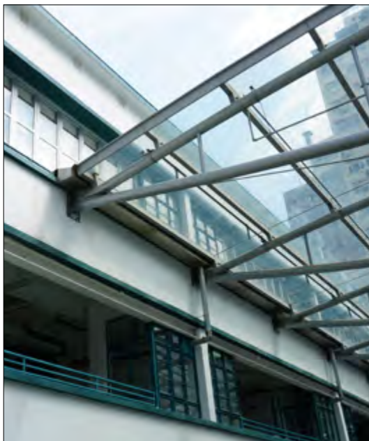
03.54 // Opposite page, left: Junction between the existing building and the new cantilevered roof structure.
