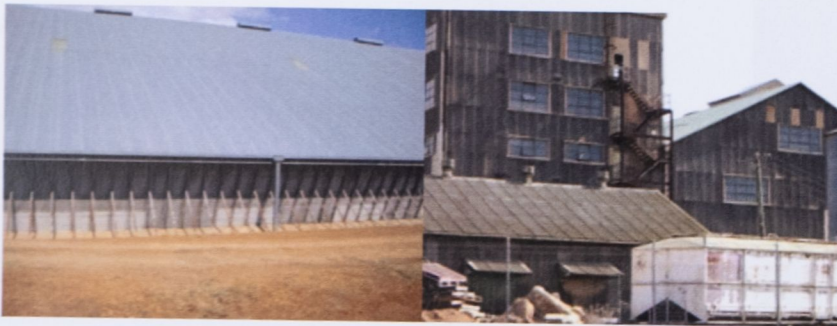
Industrial agricultural buildings_ Cowra
