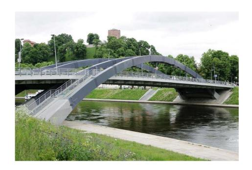
Surrounding panoramas also required protection, so this dictated a typologically original special- architectural solution for the arched bridge, which sits one hundred and one (101m) metres across the Neris River, and almost twenty metres (19.75m) in width, with three lanes of traffic flowing over it, the minimal, geometrically simple architectural masterpiece.
