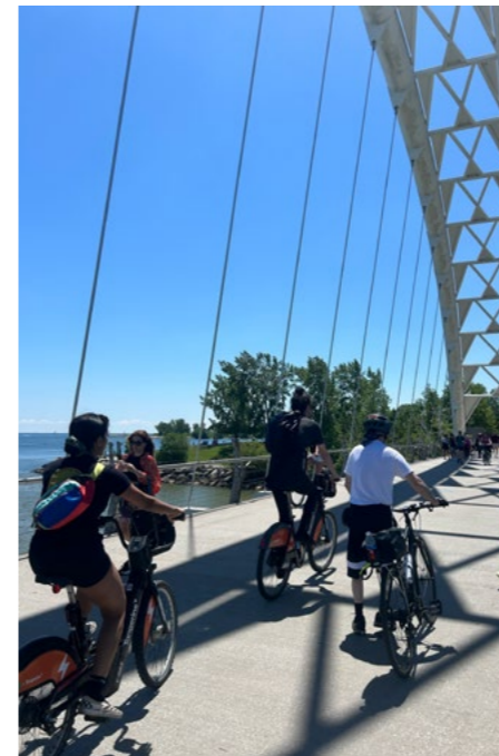
Toronto Humber Bay Arch Bridge
