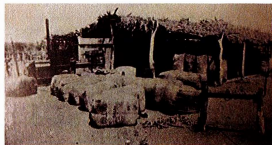
Image Right: The original shearing shed at Bullara Station. 1923. Spinifex and wire netting roof
