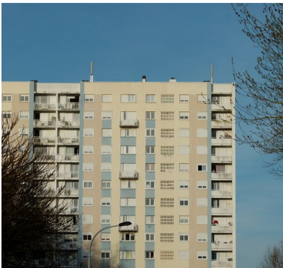
Typical Non-Refurbished Building in Estate Area
