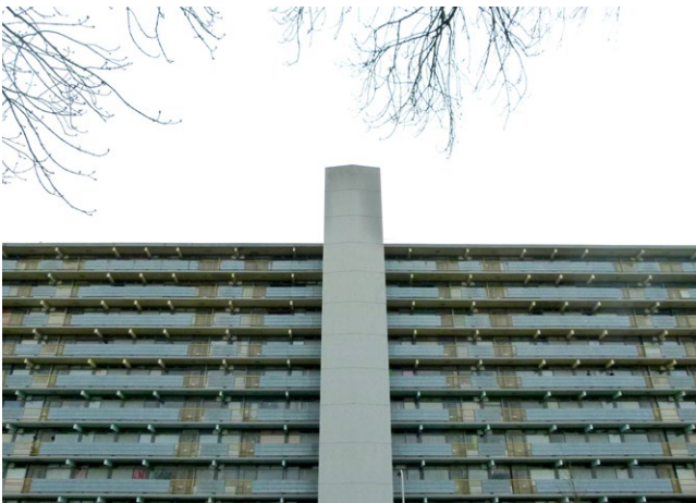
Un-refurbished Building within Estate Area
