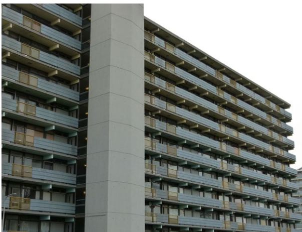
Un-refurbished Building within Estate Area
