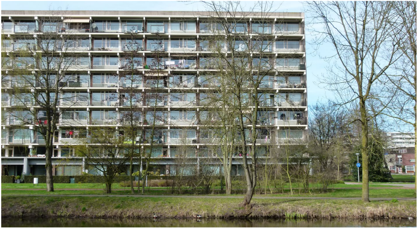
View of Refurbished Elderly Building from Surrounding
