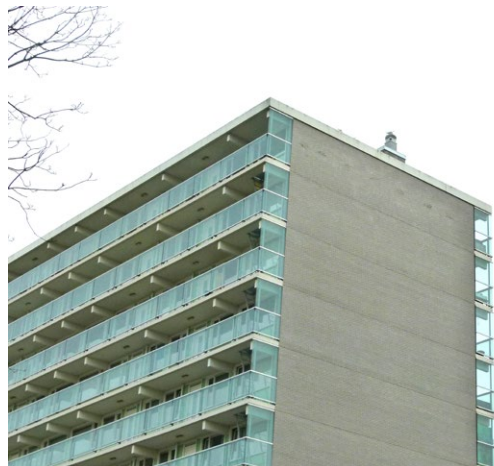
Short Facade with New Brick Wall
