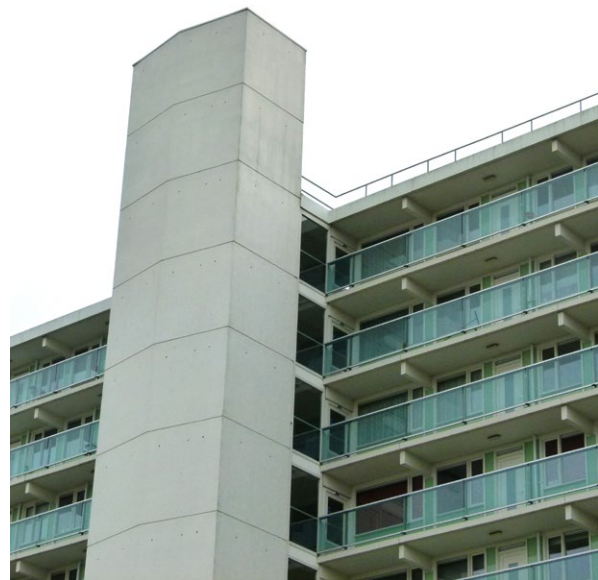
Refurbished Lift Core and Facade
