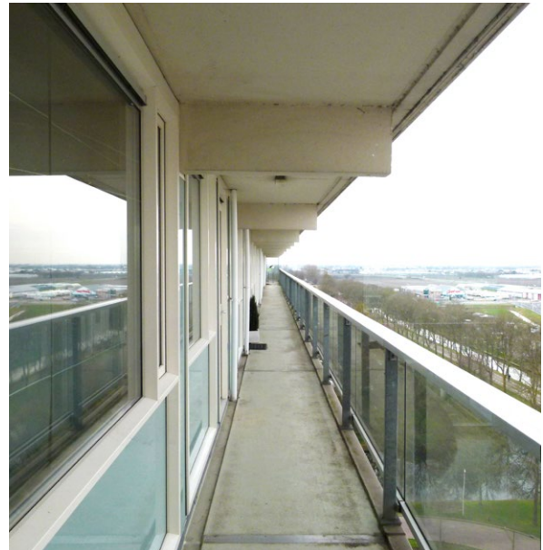
Long Deck Access with New Material Treat-
