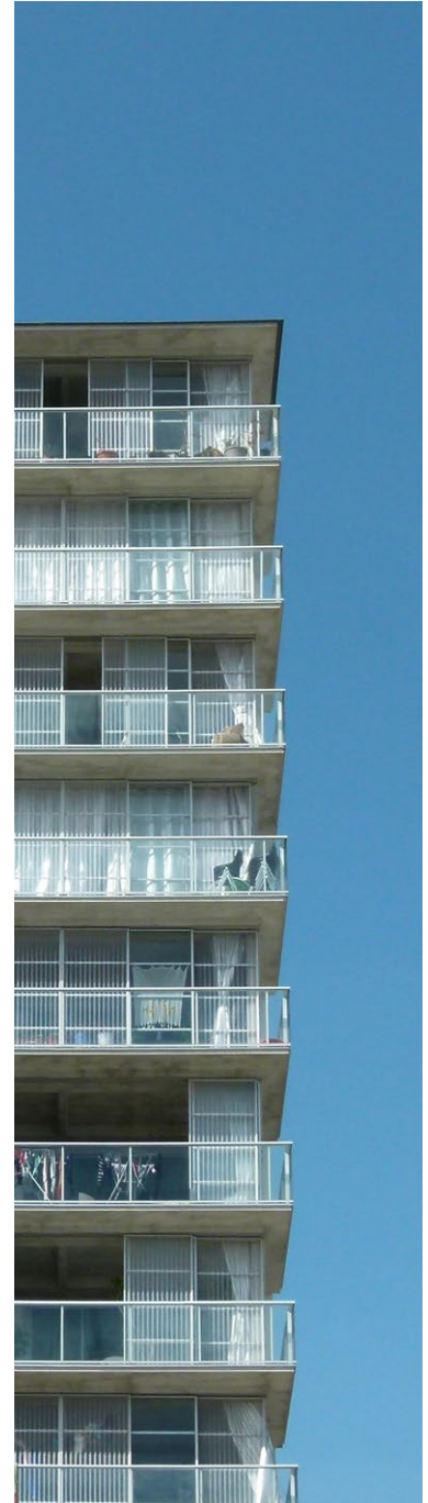
Stacked Facade, Bordeaux
