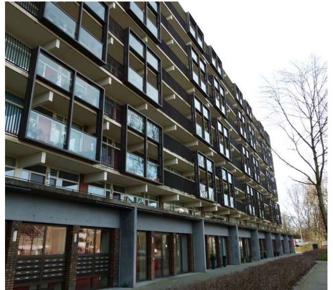
Refurbished Mixed Tenancy Building
