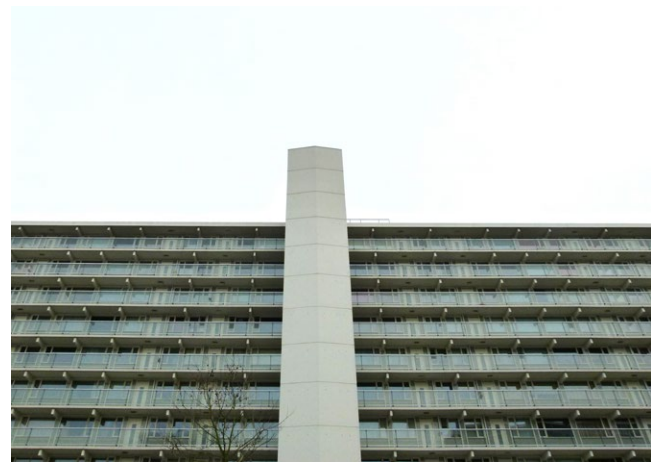
Refurbished Building within Estate Area
