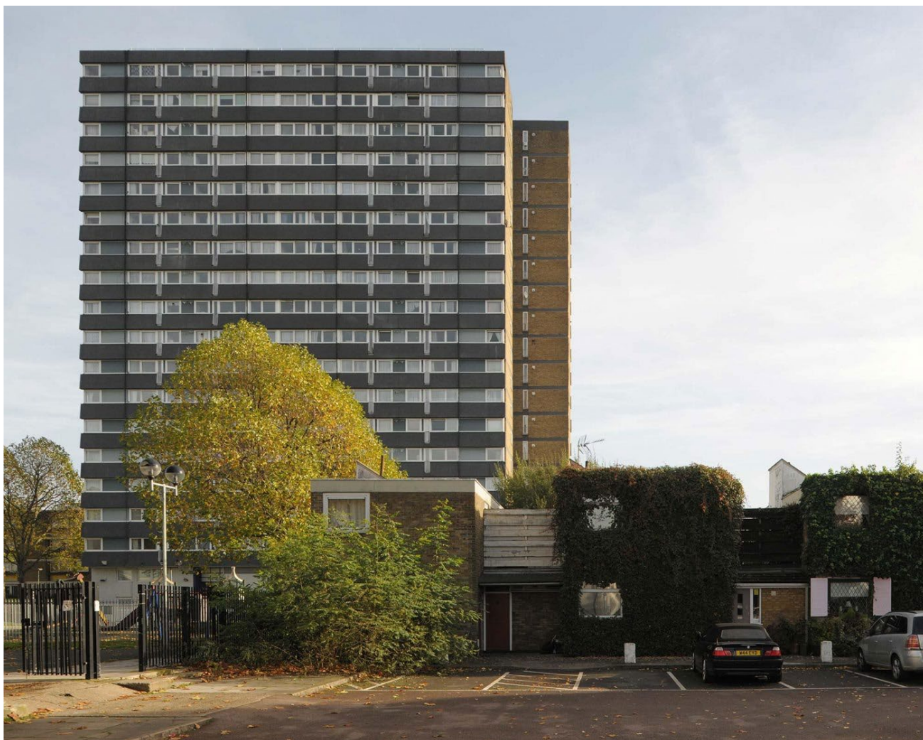
Lulworth Tower Currently (Photo Courtesy of Mae
