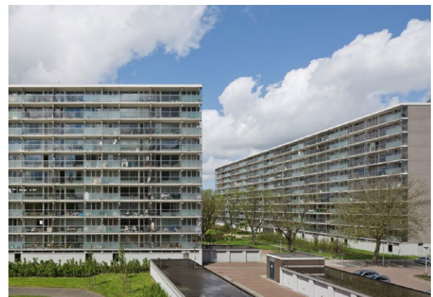
After Refurbishment (Photo Courtesy of Atelier Kempe Thill)
