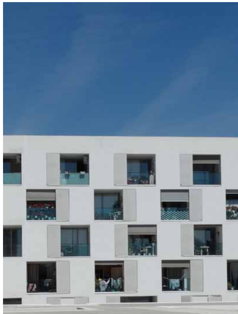
Individual balconies, Can Travi, Barcelona, Spain.
